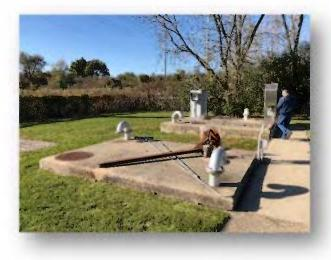
stations are constructed to pump the wastewater through force mains to higher elevations. The wastewater is then discharged to the downstream gravity sewer. The arrangement of a typical lift station is shown in Exhibit 3-4.
