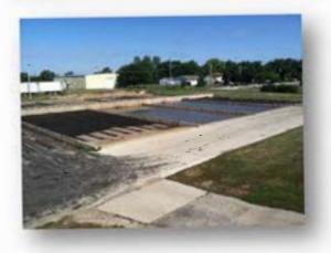
for drying bed dewatering. Although stabilized, biosolids stored on exterior drying beds may induce odors. Therefore, these would not be recommended for the Authority due to the current emphasis on odor reduction throughout the facility.
