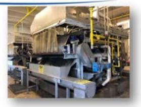
Digested sludge is routed to the Sludge Dewatering Building which houses two Belt Filter Presses (BFPs). Polymer mixing units provide polymer to the digested sludge to encourage coagulation of sludge, improving dewatering efficiency. Shaftless screw conveyors are used to carry dewatered sludge from the BFPs to trucks for removal.
