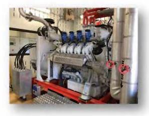
After biogas is produced in anaerobic digesters, it must be conditioned before it can be sent to CHP/cogeneration unit. This is to maximize energy efficiency of gas and preserve the mechanics of the cogeneration unit. Biogas typically has high levels of hydrogen sulfide and siloxane, as well as water vapor. These components are destructive to the cogeneration engine and if not removed can result in damage to the unit and significantly shortened service lives.
