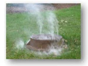
sewer system can sometimes be identified where check valves are not installed on the pump discharge
