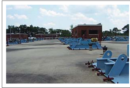
HPO basin deck
